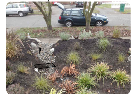
OVERFLOW AREA WITH ARMORING (VIEW FROM RAIN GARDEN)
