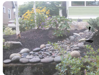
OVERFLOW AREA WITH ARMORING (VIEW FROM RIGHT-OF-WAY)
