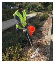
The most important times to remove debris and trash from the bioretention cell are before and after a storm. Heavy rains can cause trash and debris to collect around curb openings and overflow drains and block stormwater flow.
