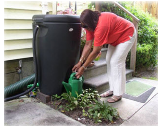
Figure 1. A rainwater harvesting system being used for watering flowerbeds
