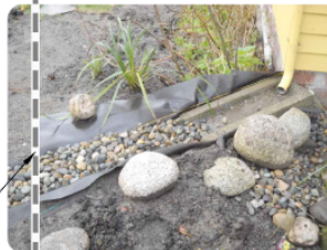
EXAMPLE DOWNSPOUT TO RAIN GARDEN ROCK TRENCH CONNECTION
