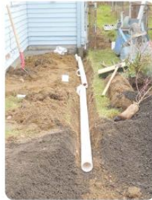
DOWNSPOUT TO RAIN GARDEN PIPED CONNECTION UNDER CONSTRUCTION
