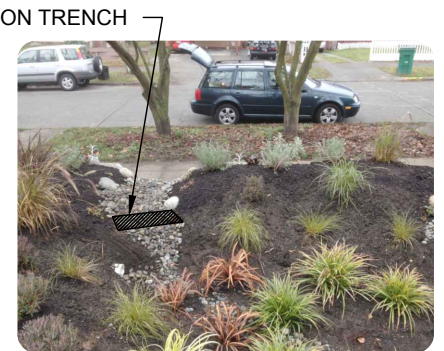
OVERFLOW AREA WITH ARMORING (VIEW FROM RAIN GARDEN)
