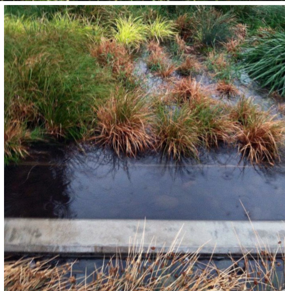
Each swale is approximately 270-feet long and up to 16 feet wide.
