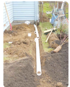
DOWNPOUT TO RAIN GARDEN PIPED CONNECTION UNDER CONSTRUCTION
