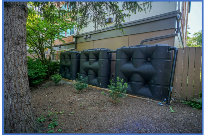
Three 530-gallon cisterns on north side of building.
