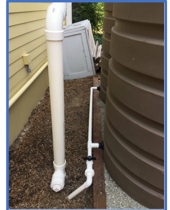
Building 3 Two 420-gallon Bushman cisterns with overflow to side sewer.
