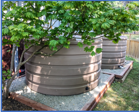
Building 1 Two 1,320-gallon Bushman cisterns with overflow to side sewer.
