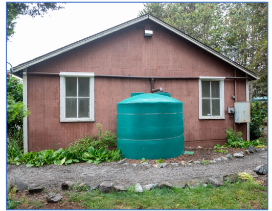
The six cisterns can hold a capacity of 16,500 gallons.
