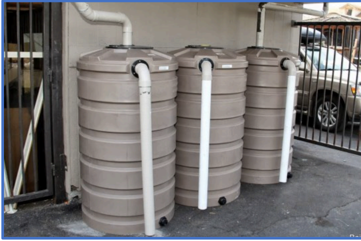
Three 205 gallon cisterns capture 2,106 ft 2 of roof area and overflow into a catch basin located in the apartment courtyard.
