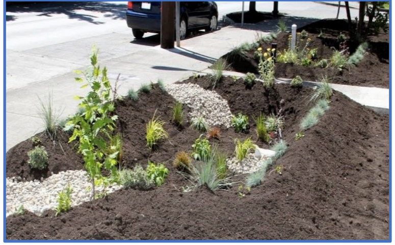
3,730 ft 2 of roof area is captured by two rain gardens, with one with overflow to the side sewer and the other overflows to the sidewalk.
