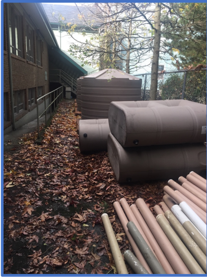
Cisterns and new piping unloaded and ready for the installation process to begin.
