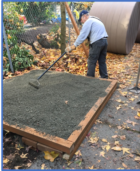
Rain Dog Designs prepares the base that will hold one of the 1,320 gallon cisterns.
