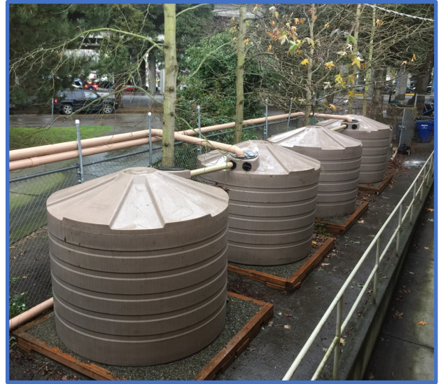
These four 1,320 gallon cisterns capture 5,920 ft 2 of roof area while the three "Slimline" cisterns capture 1,762 ft 2 of roof area.
