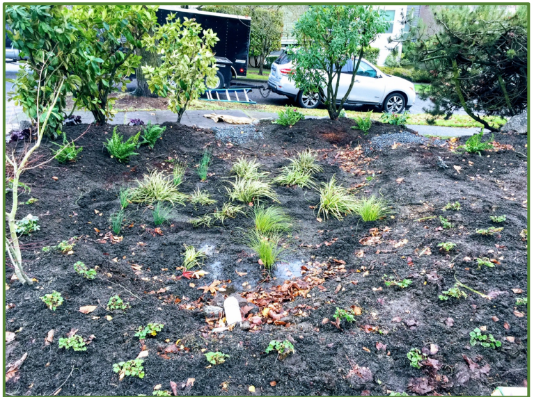
Newly installed rain garden after a heavy rain.
