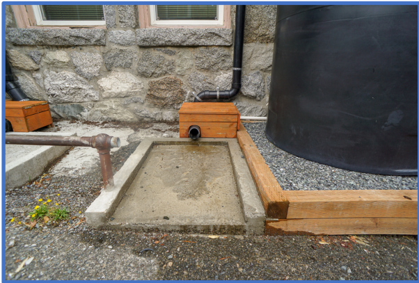
The cisterns overflow to the alleyway.
