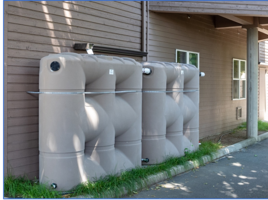
Two 530-gallon cisterns side by side capturing the large roof.
