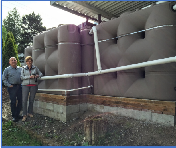
RainWise Contractor Rain Dog Designs installed the four 530-gallon “slimline” cisterns.
