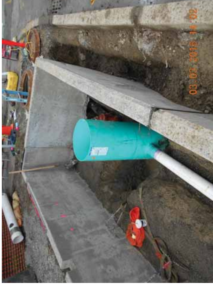
Delridge Piped underdrain to UIC well
