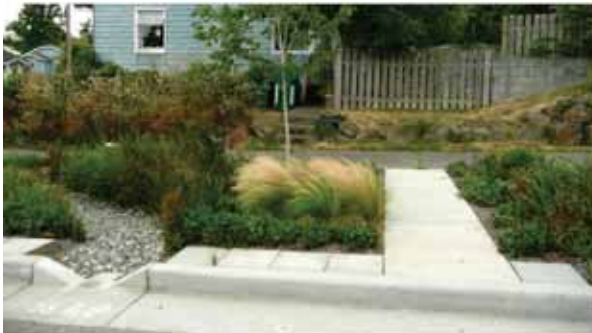
Access path is within 15' of parcel path at graded facility. Acceptable.
