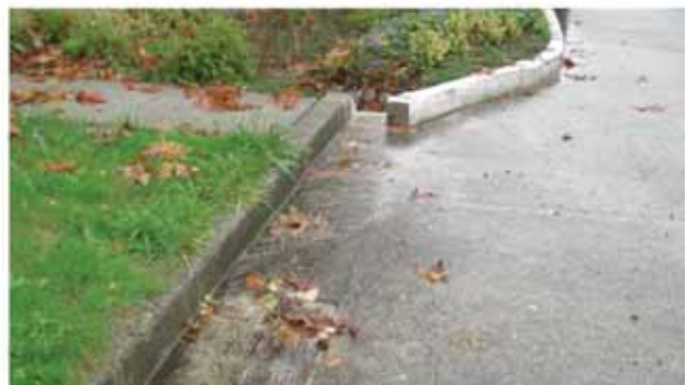
Street gutter flow into curb bulb drain curb cut
