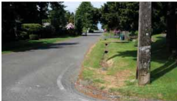
Existing ditch conveyance
