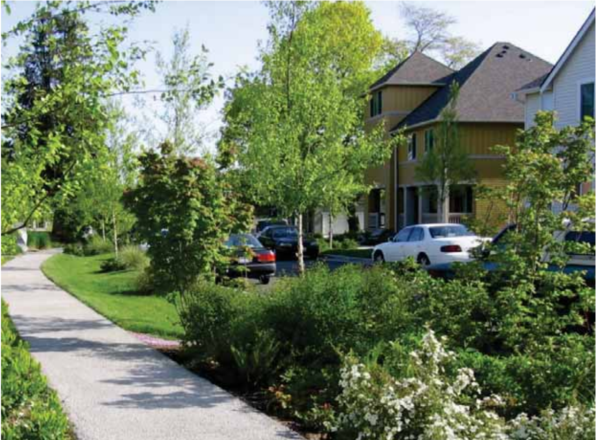
Image: Bioretention cells (grass and vegetated) with elevated underdrain after several years of plant establishment (High Point neighborhood).
