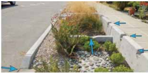
Concrete and cobble splash pad meets COS Std. Plan 295b
