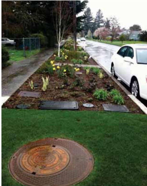
UICMH is labeled “Property of King County” and “UIC Drain” to differentiate it from typical MH
