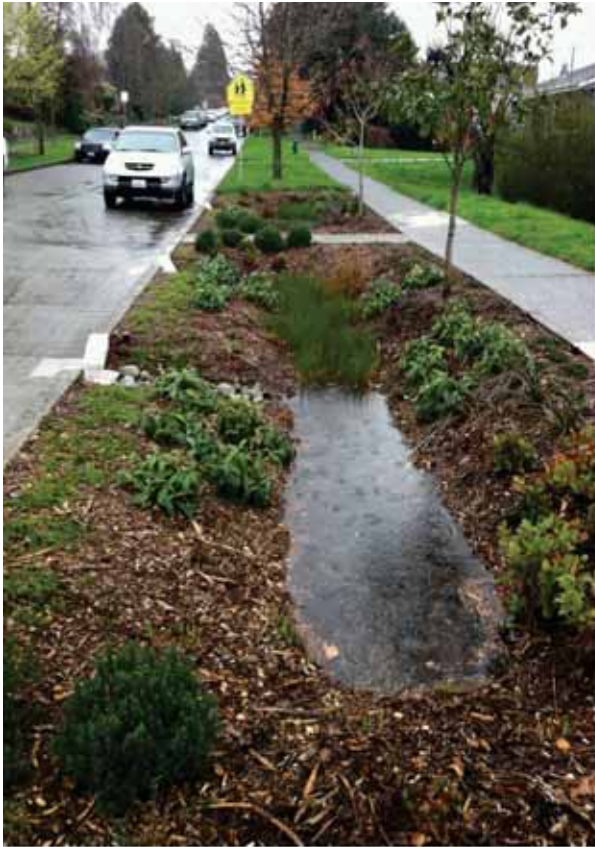
Bioretention with sloped sides on Neighborhood Yield, COS Std. Plan 293a. First winter season.
