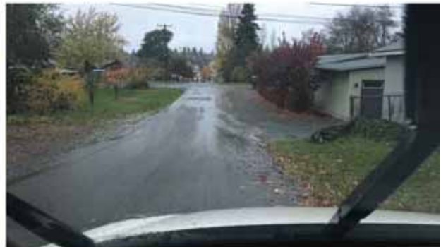
Sheet flow transition along curbless street length
