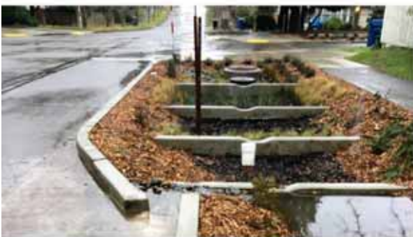
Review need for weirs and total number and provide wider intervals
