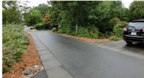
Curbless facility with narrow road, perpendicular parking bays, sidewalk on one side, notice rock pockets to protect edge at driveways, 2nd Ave NW
