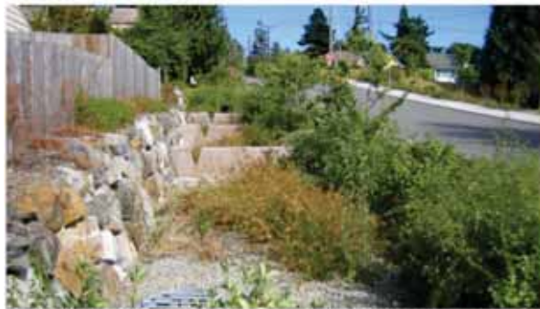
Constrained. Access zone not provided for fence maintenance and vertical drop at property line.
