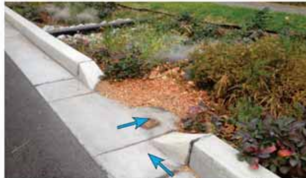
Drain curb cut is too wide for urban condition and cars may park partway in cell.
