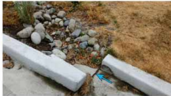
Drain curb cut does not meet COS Std. Plan 295d. Missing vertical drop from gutter to top of bay. Curb alignment and design not per standard.
