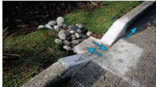
Secondary drain curb cut meets COS Std. Plan 295c.
