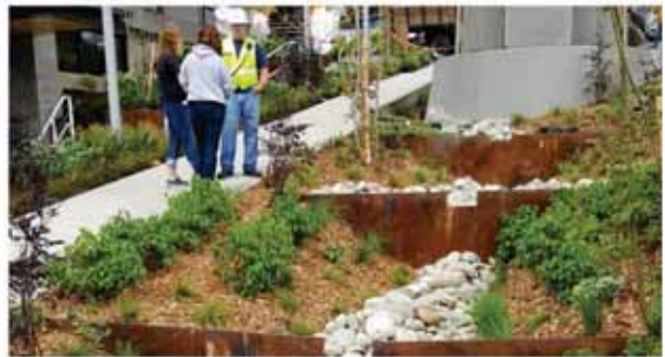
Corten steel weirs example. Recommended top edge, especially sidewalk edge, be treated (such as round molding) to avoid sharp edges
