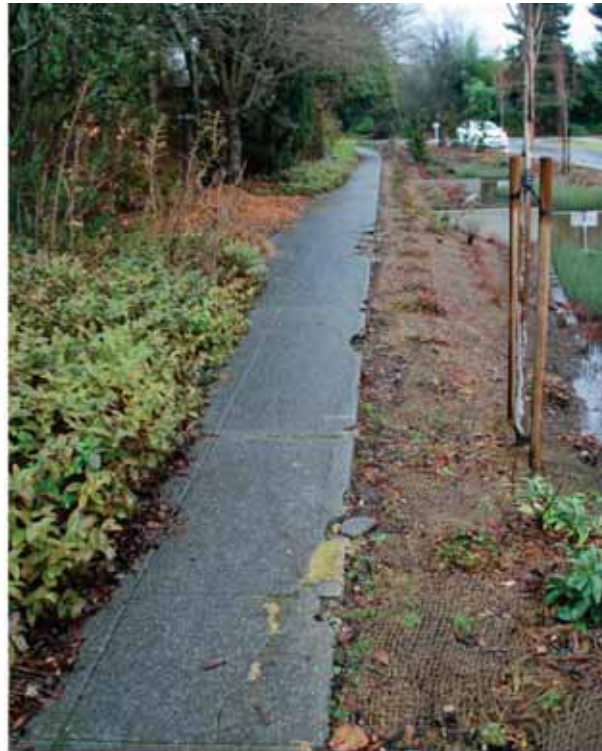
Sidewalk requires replacement and trimming of vegetation overgrowing sidewalk.
