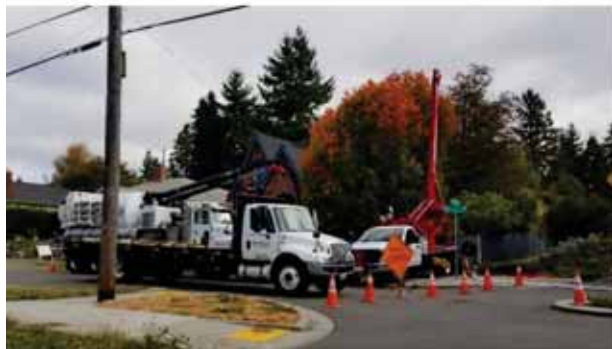
Support truck, drill rig, vector truck, and traffic
