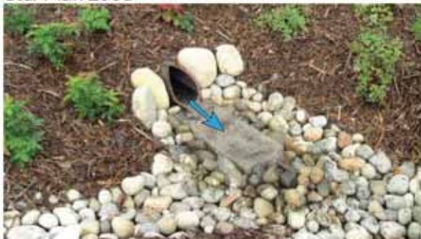
Concrete splash pad at pipe discharge point meets GSI detail B-5A in Appendix D. First winter season.
