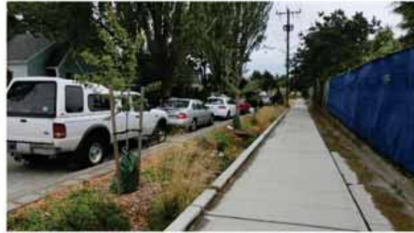
Length of facility too long without a crossing path. Not recommended. Requires special review.
