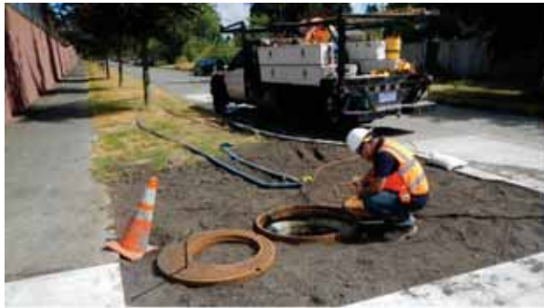
UMH easily accessed away from bioretention. Preferred.
