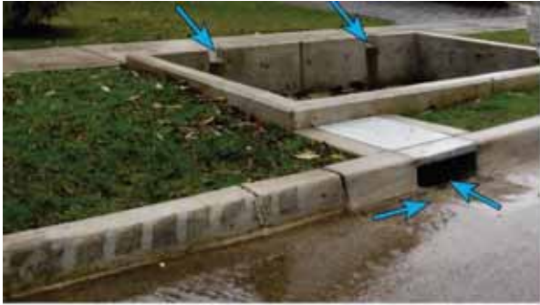
Enclosed drain curb cut. Lid too heavy for removing and resetting. Provide holes on all four sides for lifting lid.
