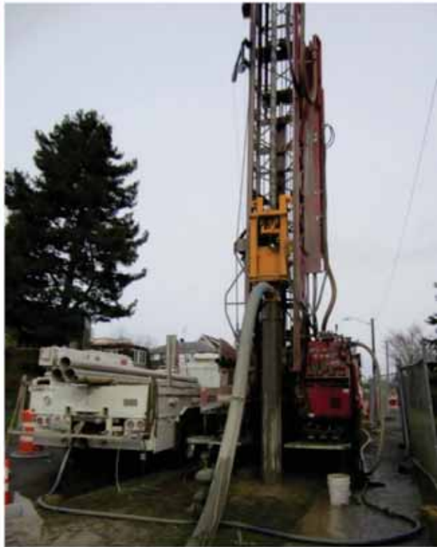
Larger rig used to drill UIC wells
