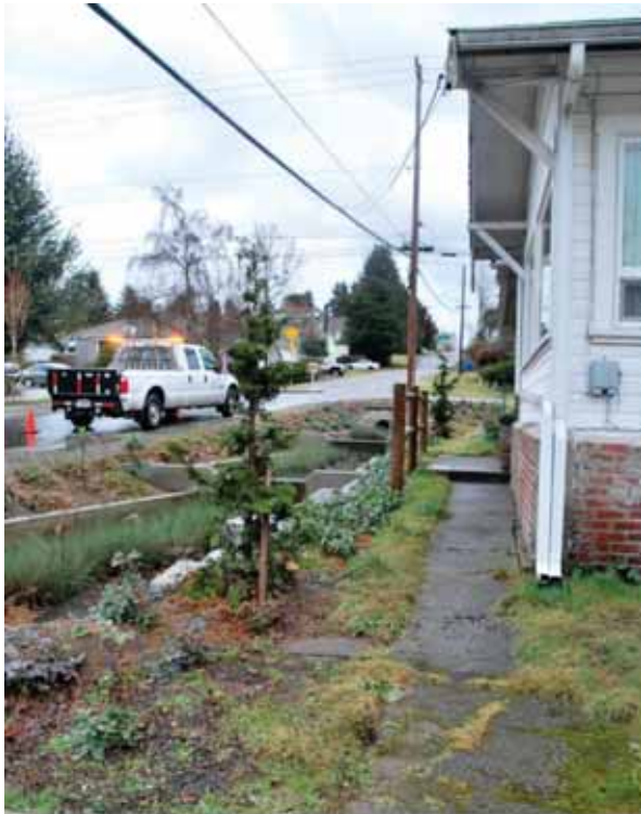
Constrained. Small lawn strip left for parcel owner to maintain. No level access along property line. Fence rail for vertical drop at parcel access with steps.
