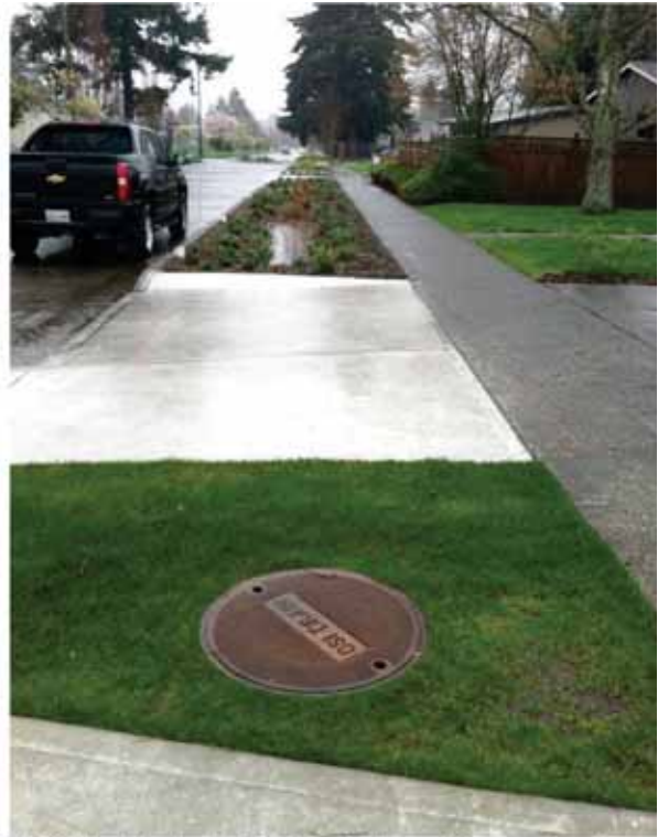
UMH is labeled "GSI Drain" to differentiate it from typical MH
