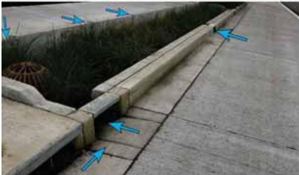
Continuous curb top. Narrow width allows for rake to clean out curb cut from sidewalk.
