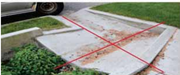
Oversized curb cut is not appropriate for urban streets. Does not meet standard plans and excess hardscape impacts access.
