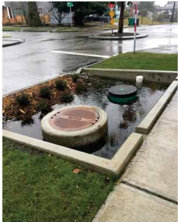
Maintenance hatch not easily accessed due to weight of lid and location within a walled area. Placement in cell reduces infiltration area. Not recommended.
