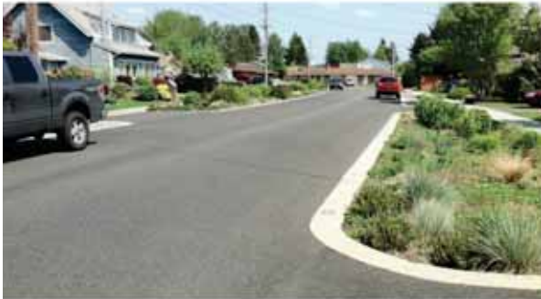
Curbless facility with parking on both sides, notice plants up to road edge and no step out zone, 8th Ave, Puyallup
