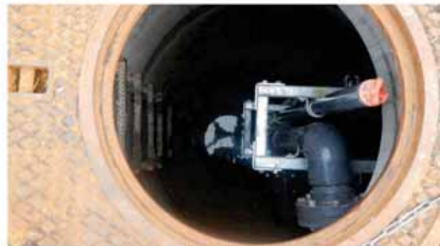
UIC maintenance hole with UIC assembly and observation port accessible at MH openings.
