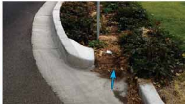
Drain curb cut at curb bulb. Curb alignment does not meet Std. Plan 295d.
