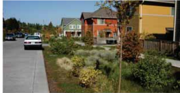
Curbless facility with parking on both sides, 32nd Ave SW, Seattle
