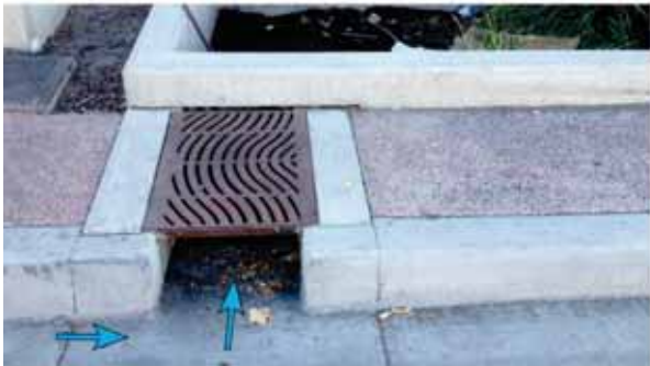
Enclosed drain curb cut with planter. Holes not sized for lifting lid for cleaning.
