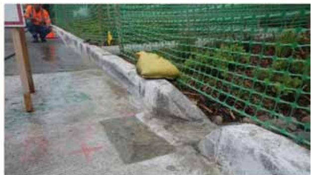
Gutter flow testing during construction
