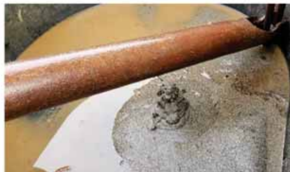
Sand pumped from UIC during rehab
