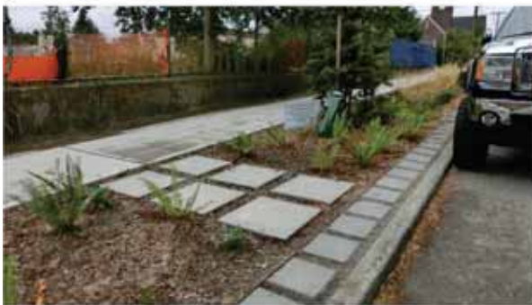
Paver access path. Not recommended. Requires special review.
