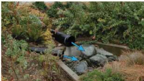
Pipe discharge with energy dissipation downstream of presettling vault (not shown). Custom design for managing flows from multiple blocks. Too much exposed pipe.
