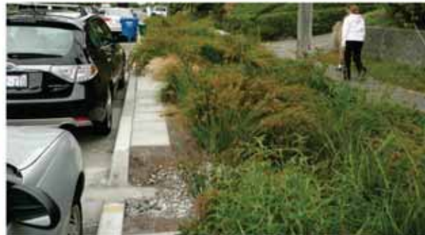
Tight pavers step out zone after installation
