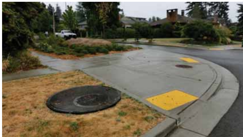
Image: Presettling MH with dual opening sizes and located in level area for MH access. Structures located outside ADA ramp and landings. Photo from SPU's Venema project.
