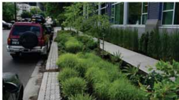
Paver step out zone - difficult to weed
