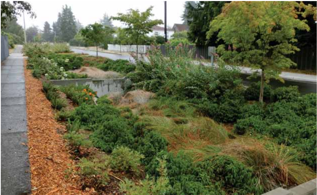
Image: Full ROW retrofit for SPU's Venema project along a Neighborhood Curbless street. Photo shows the various planting zones starting from existing sidewalk to side slopes of bioretention cell to bottom of facility. This facility manages flow from multiple blocks.
