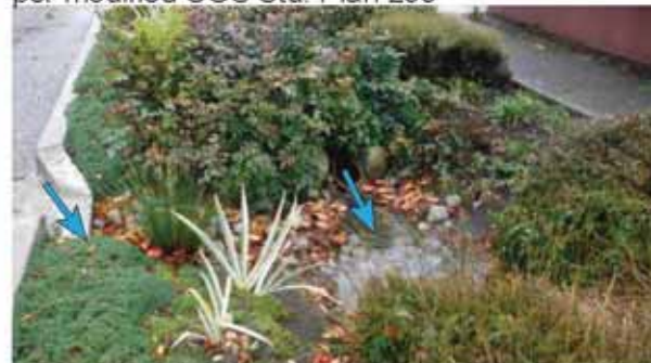
Concrete splash pad at pipe discharge point meets GSI detail B-5A in Appendix D. Third winter season.
