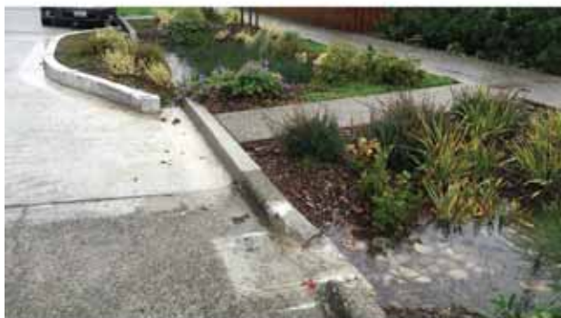
Street gutter flow into drain curb cut
