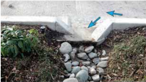
Primary drain curb cut meets COS Std. Plan 295b.
