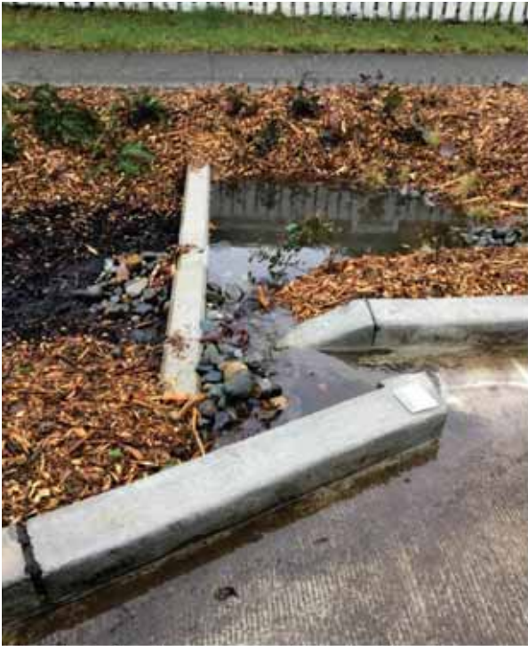
Weir location too close and block flows from curb cut. Not recommended.
