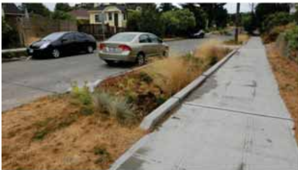
Cell with graded side slopes and a vertical wall with soil cells under walk (non-standard), suggest a stronger transition at facility ends, Ballard Phase 2
