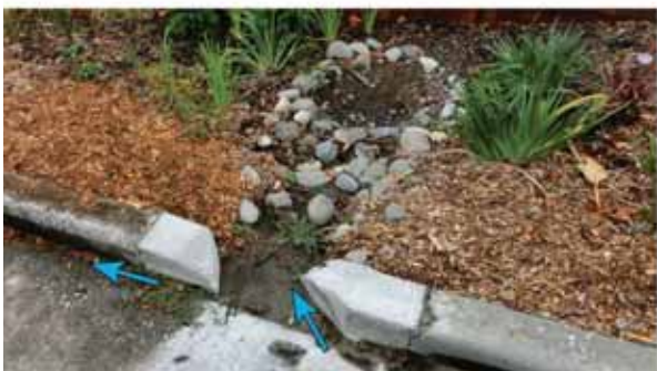
Drain curb cut does not meet COS Std. Plan 295b. Cobbles extend across bottom of cell and curb transition not per standard.
