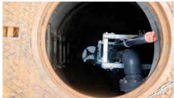
UIC maintenance hole with UIC assembly and observation port accessible at MH openings.
