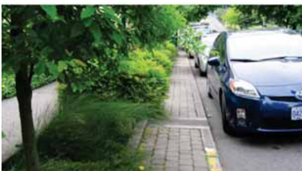
Paver step out zone - difficult to weed
