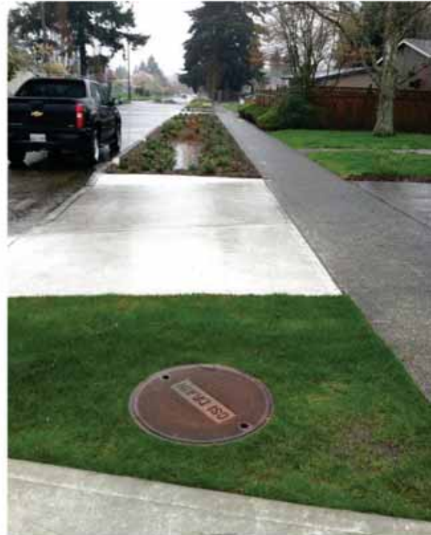
UMH is labeled “GSI Drain” to differentiate it from typical MH
