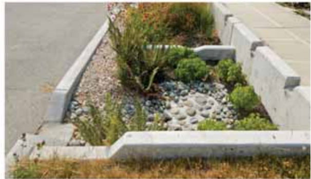
Bioretention with 3-sided wall and remaining side sloped. End walls not recommended.
