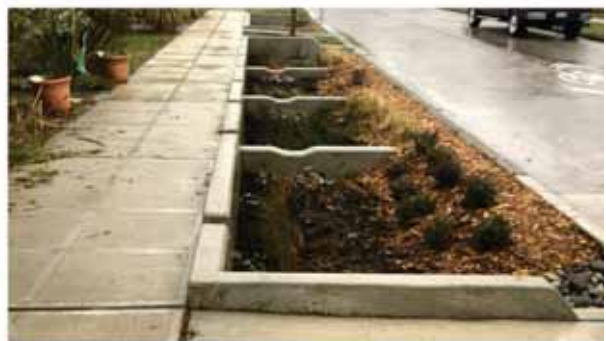
Review need for weirs and provide wider intervals
