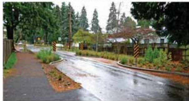
Curbless facility with curb bulbs, 17th Ave NE, Shoreline
