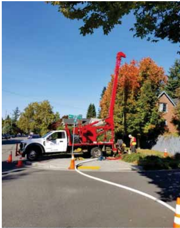
UIC Screen Well Rehab at SPU's Venema NDS
