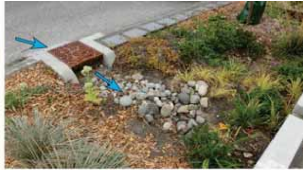
Partially enclosed drain curb cut is difficult to clean. Holes not sized for removing lid to clean out debris.
