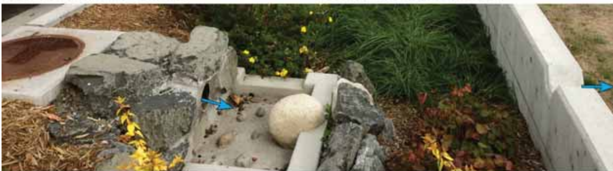
Non-standard drain curb cut. Excess hardscape, uneven, and impacts infiltration area.
