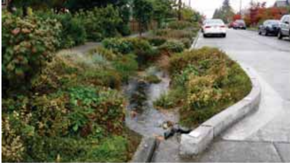
Bioretention with graded side slopes in new curb bulb during rain event, notice retrofit curb
