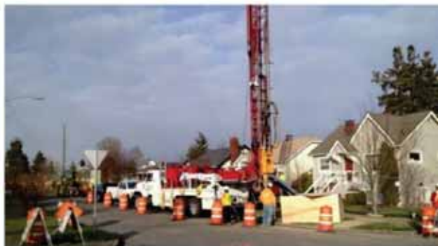
Larger rig used to drill UIC wells
