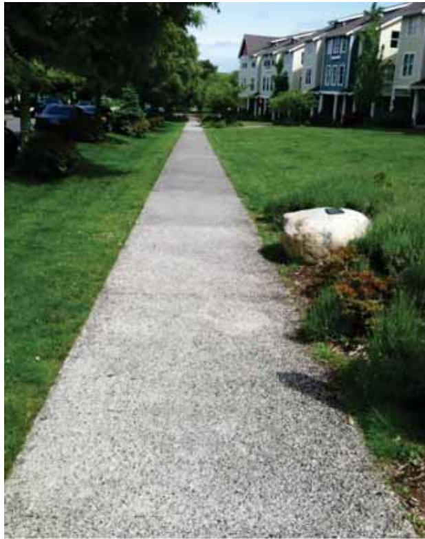
Pervious concrete sidewalk
