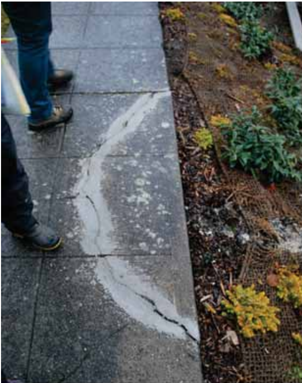
Substantial sidewalk repair adjacent to new bioretention facility.
