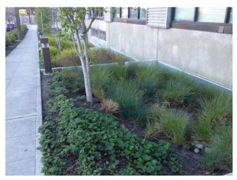
Image: Bioretention at the Goodwill building in the City of Seattle
